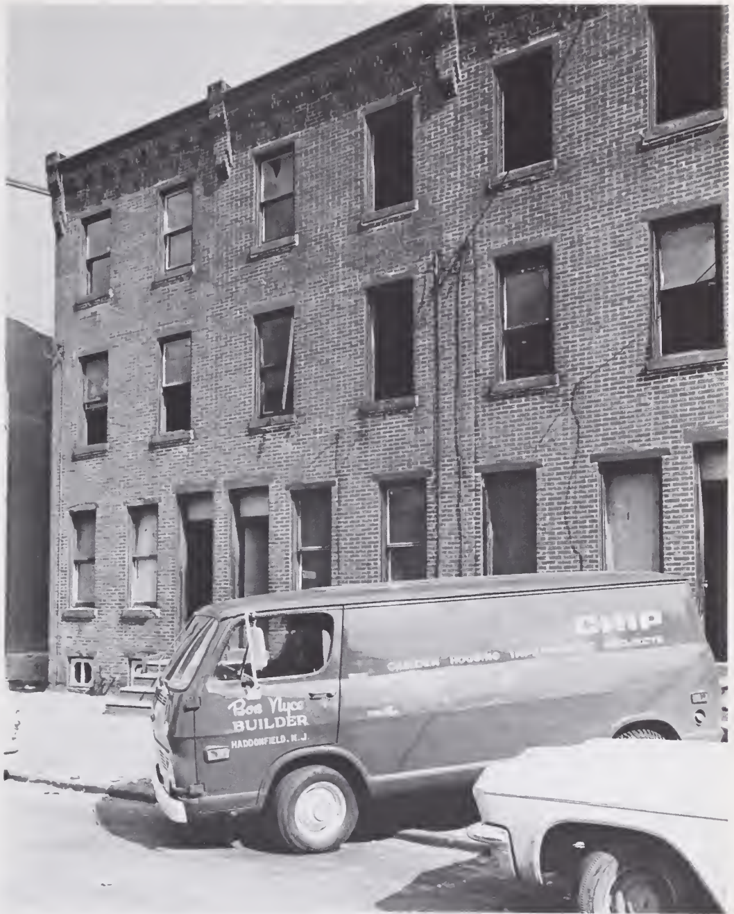
TYPICAL CONDITION OF PROPERTIES PURCHASED BY CHIP
